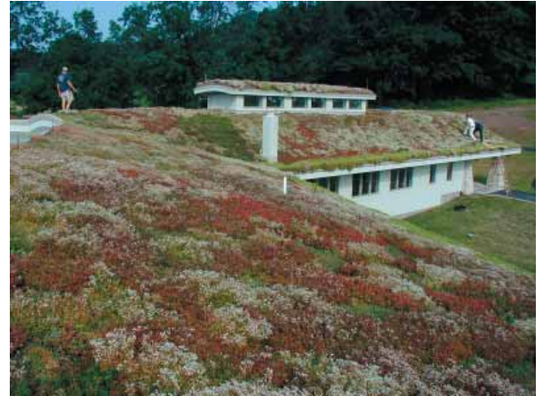
Extensive Green Roof
