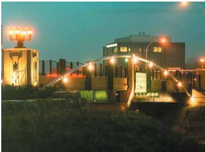
Figure 4: Burnsville Parkway Bridge
