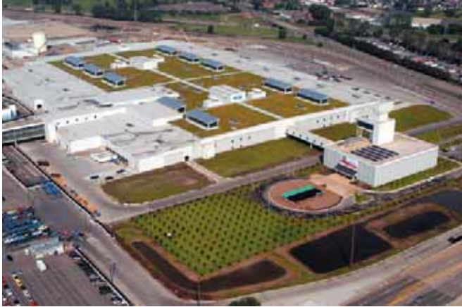
Extensive Green Roof
