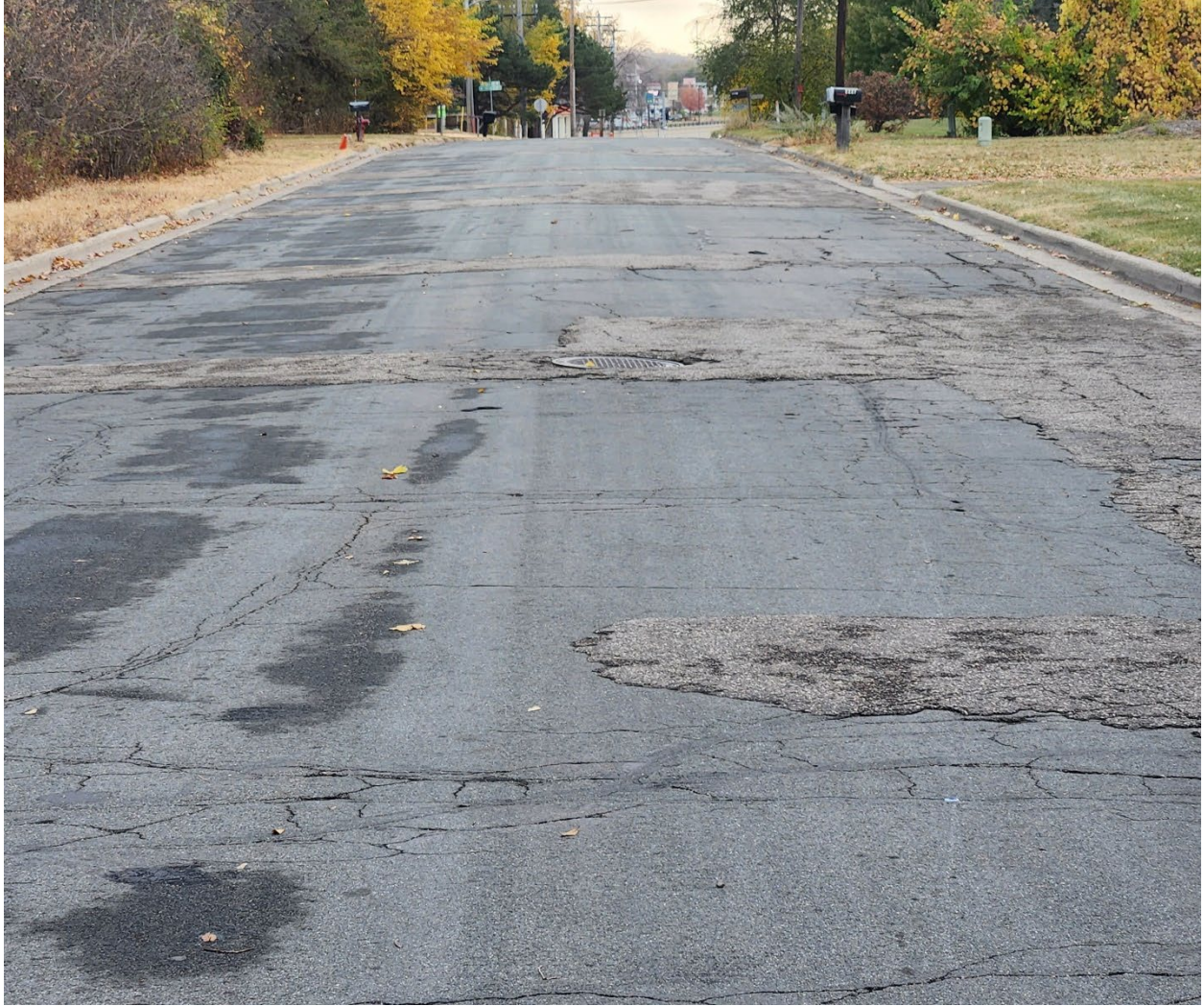
Old County Road 34, midblock, looking east at Morgan Avenue South
