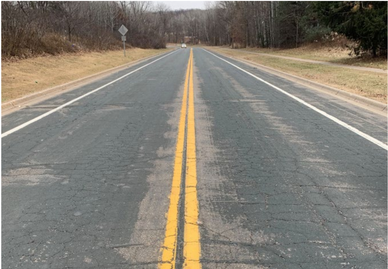
Burnsville Parkway East at County Road 11 looking east
