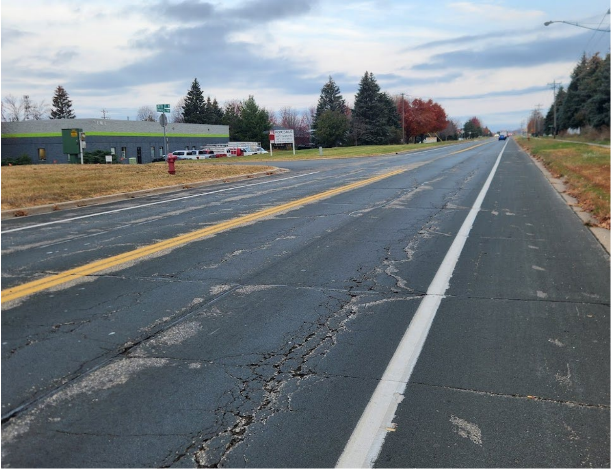
Burnsville Parkway West, looking north just south of 145th Street
