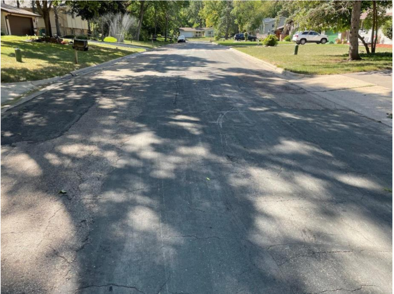
Woodview Lane looking south to Woodview Dr
