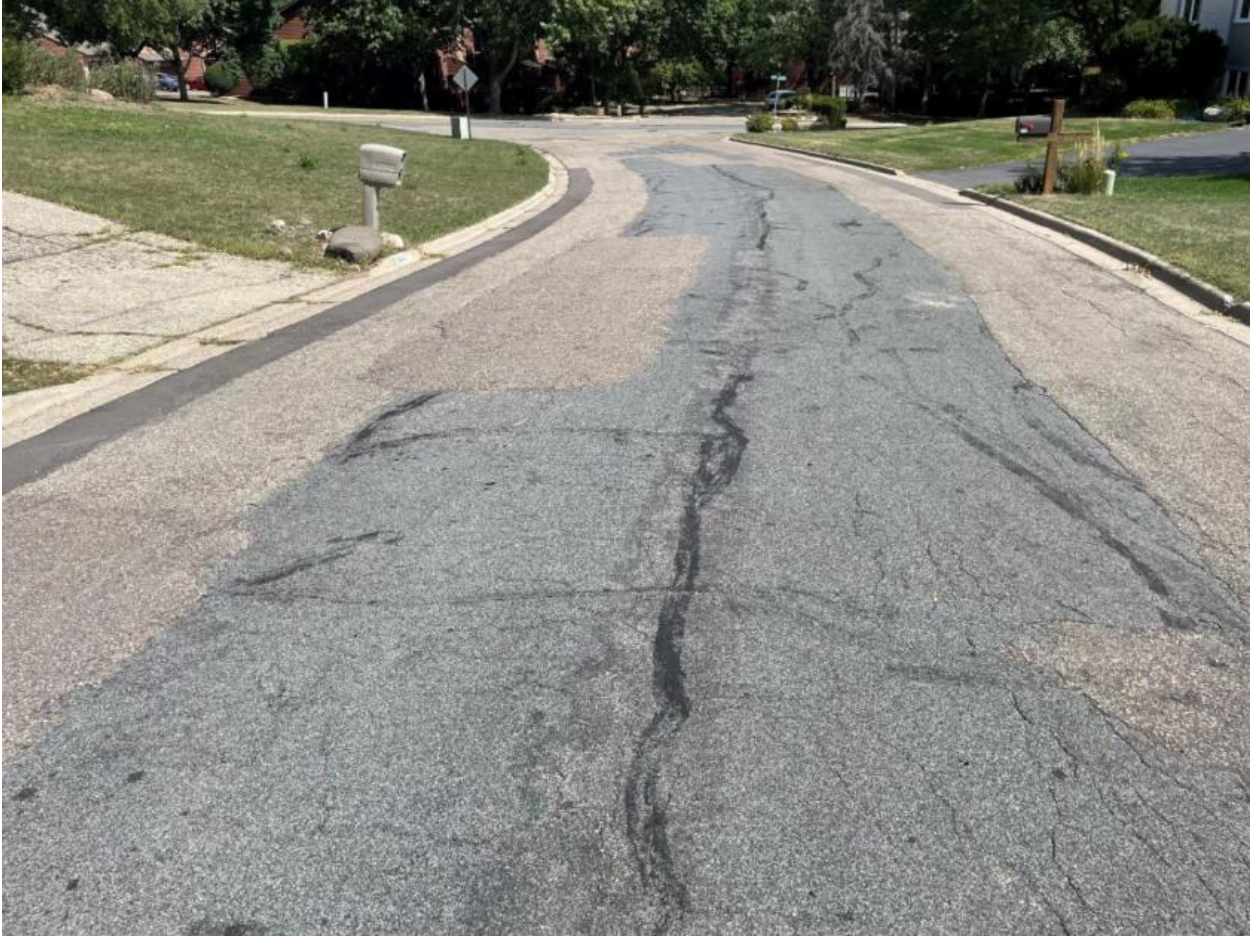
Raymar Court looking east to Morgan Avenue S
