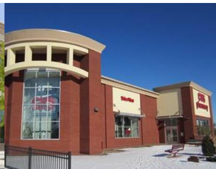
Defined base and top of building using window and door openings, and building materials.
