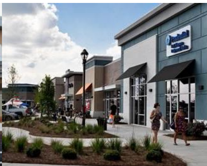
Variable façade depths, changes in materials, and awnings to create distinct modules.
