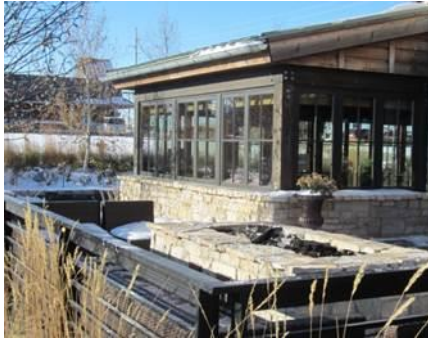
Gathering spaces, complimented by landscaping, decorative fencing and lighting.
