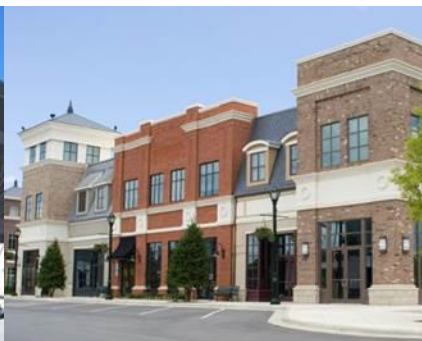
Ground level building accents. Defined middle and top of building using changing materials, windows, roof design, etc..
