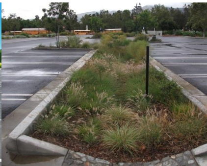
Planted landscape islands for beauty and to treat stormwater runoff from parking areas.
