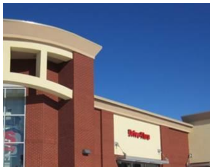
Variety in roofline height and design. Corner roof emphasizes front entry. Attractive cornices.
