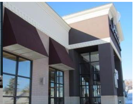
Defined horizontal and vertical modules using building materials, awnings, and windows and doors. Projected windows.
