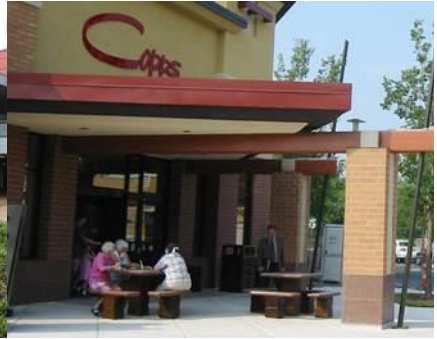
Entry plaza with accessible public seating and dining areas.
