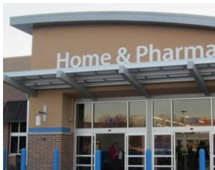
Variable façade depth, defined roof line, windows and doors at base level, and changes in materials. Use of canopies.
