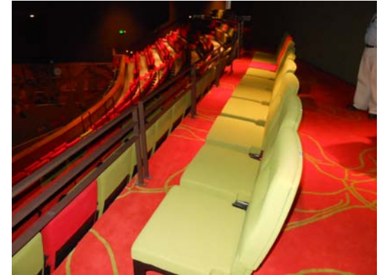
Photo 3: View of wheelchair positions in auditorium. The chairs can be removed or used as companion seating.
