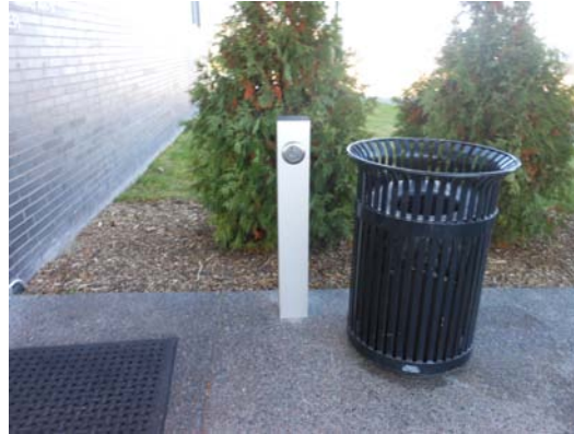
Photo 2: Relocate the trash can so it does not obstruct access to the power door opener.
