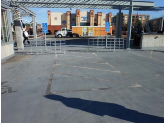
Photo 1: View of accessible parking. Accessible parking spaces with 8' wide aisles are provided throughout the parking facilities.
